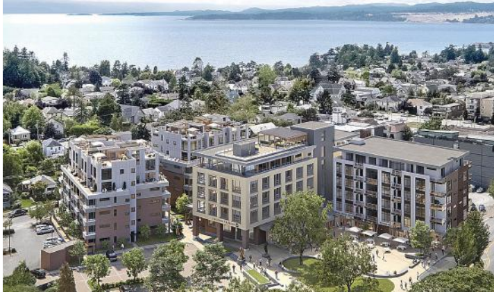
Esquimalt Town Square Construction Moving Forward Aragon Properties Ltd. | (PC: Western Investor)
