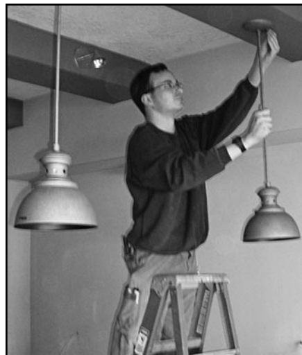
Apprentice, Brian Phillips working on the Bear Mountain Condo Project.
